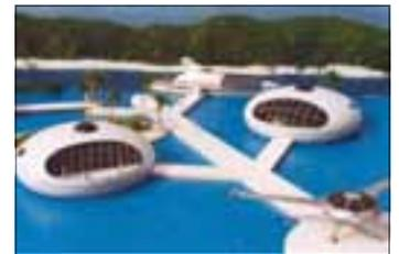
Homes are prefabricated from a new type of pre-stressed reinforced concrete with a flexible ceramic external coating; they are relatively maintenance-free, fireproof, and impervious to weather. Their thin shell construction is mass-produced in a matter of hours. With this type of construction, there is minimal damage from earthquakes and hurricanes.
