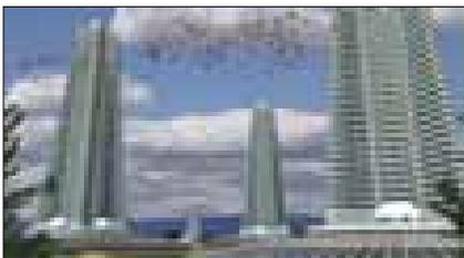
These skyscrapers are constructed of carbon fiber-reinforced and pre-stressed concrete. They are stabilized against earthquakes and high winds by three massive, elongated, tapered columns, which are 100 feet wide at the base. This tripod-like structure is reinforced to diminish compression, tension, and torsion stresses.
